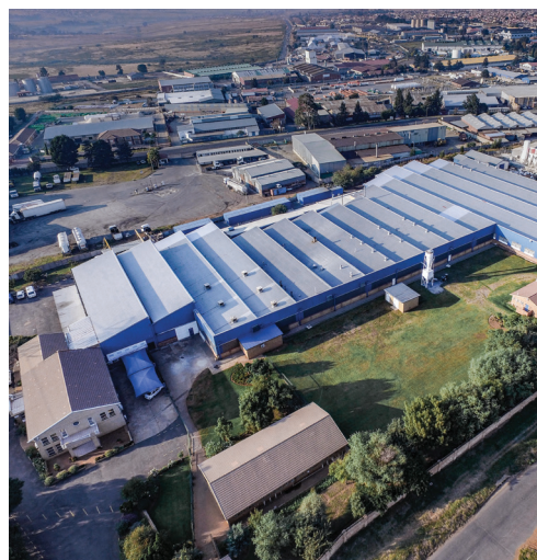
Grinding Techniques headquarters in Chamdor (Krugersdorp)
